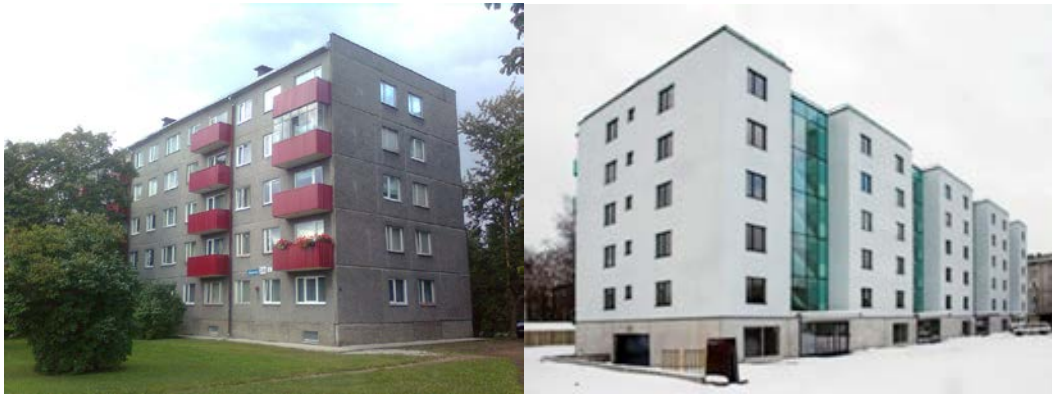
Figure 1 Examples of analysed building (old (left) and new (right)).
