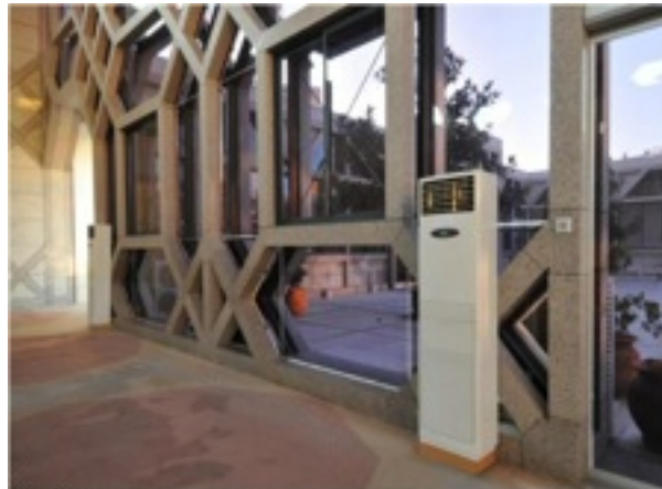
Figure 2 - Temporary Air Conditioning Units
