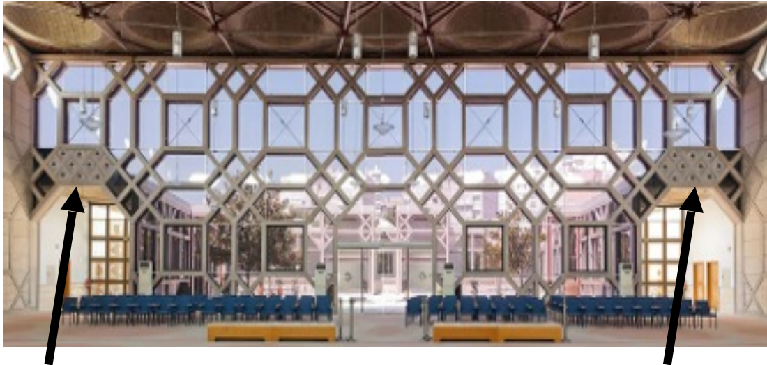
Fig 19 Proposed arrangement that will allow appropriate supply air distribution, as indicated by CFD.
