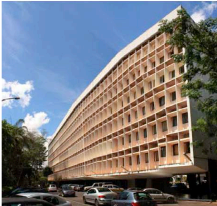
Figure 7. SQS 108 Block E, North East elevation (the cobogó elevation) (top) and the South West elevation (the brise soleil elevation) (bottom) Source: (Author, M S. Franco)
