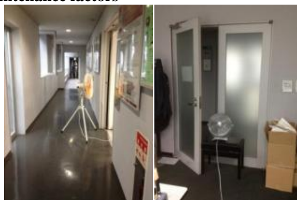
Figure 12. Opening the ventilating doors into the thoroughfare passage ways directly affected privacy; Vertically pivoted windows in the ventilating corridor obstruct free movement of people.
