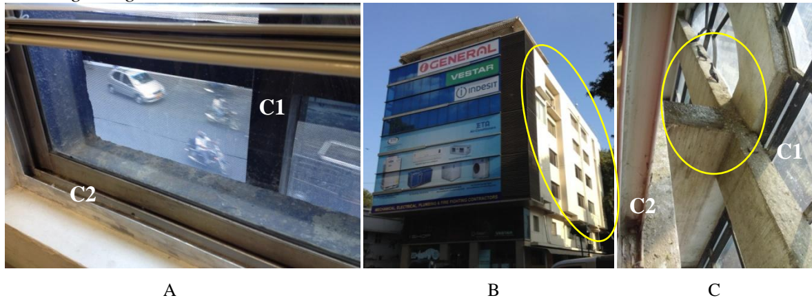
Figure 10. Windows inside made inoperable and ineffective by curtain glazing and bird breeding. (A, B) Interior and exterior views of the cosmetic curtain glazing layer and (C) Avian breeding and debris collection between the exterior curtain-glazing (C1) and the operable window (C2);. (B1) Balcony spaces being merged with the office interior space often in violation of the local by-laws, making window operation less than promising
