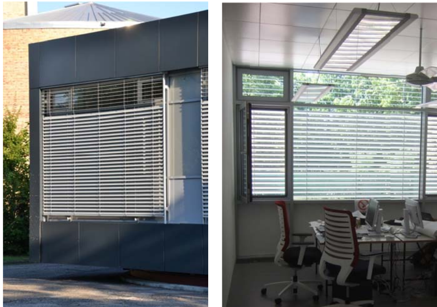
Figure 3. Venetian blinds with daylight guidance
