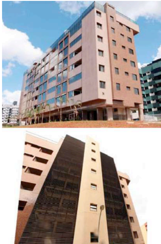
Figure 10. SQN 109 Block N, North East elevation (top) and the South West elevation (bottom) Source: (Author, M S. Franco)
