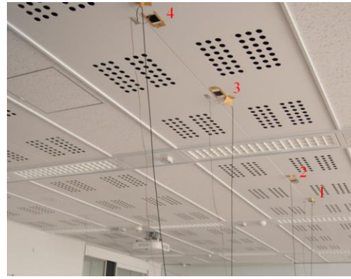
(b) Radiant ceiling panel system and sensors
