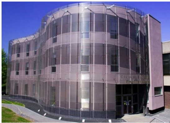
(a) Case study building
