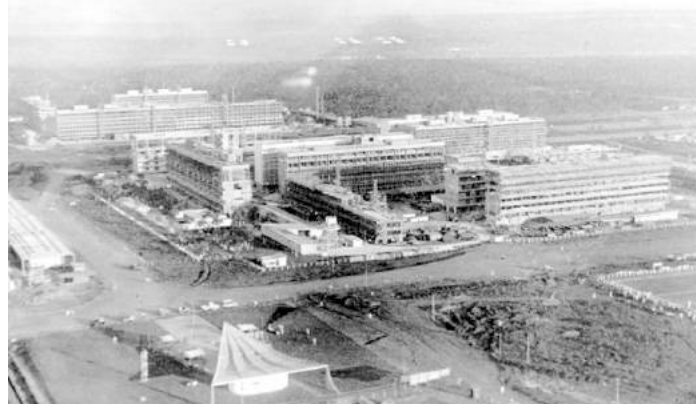
Figure 4. Superblock South (SQS) 108 under construction Source: (DesignKULTUR, 2013)
