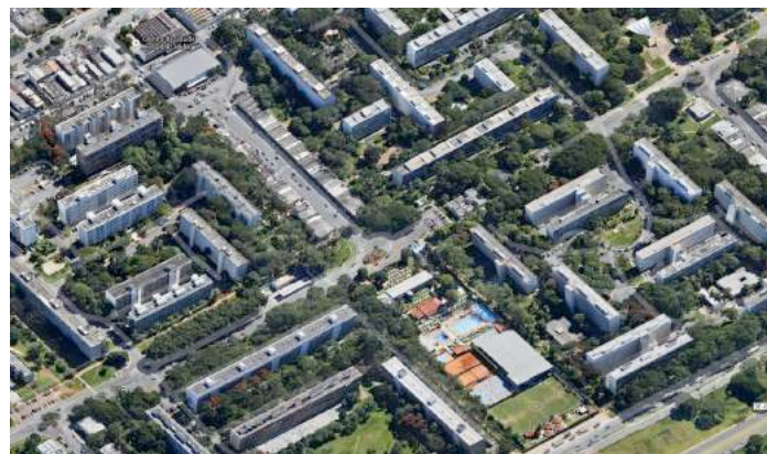
Figure 5. Superblock South (SQS) 108 today. Source: (Google maps)
