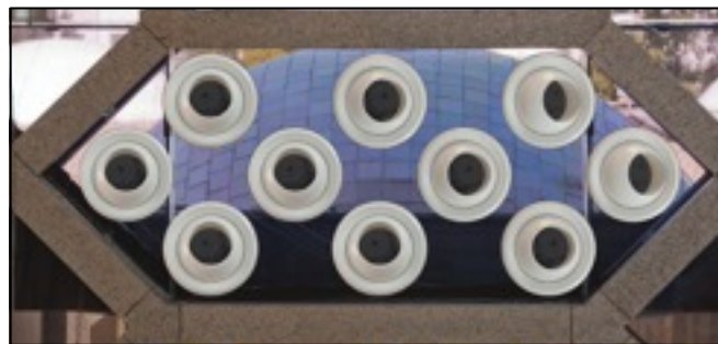
Fig 20 - Mock up of "injector" type supply air outlets.
