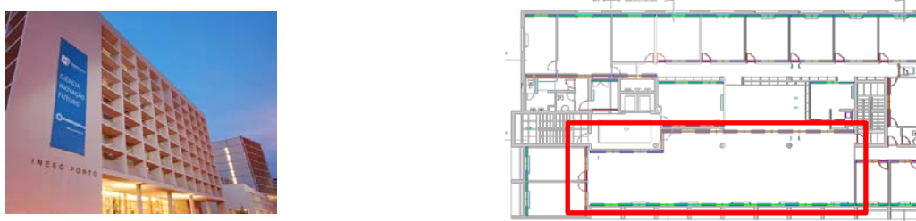
Figure 4. INESC façade of old building and layout
