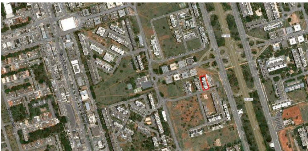
Figure 11. Aerial view of SQN 109 with Block N highlighted, showing the lack of established vegetation Source: (Author and Google maps)
